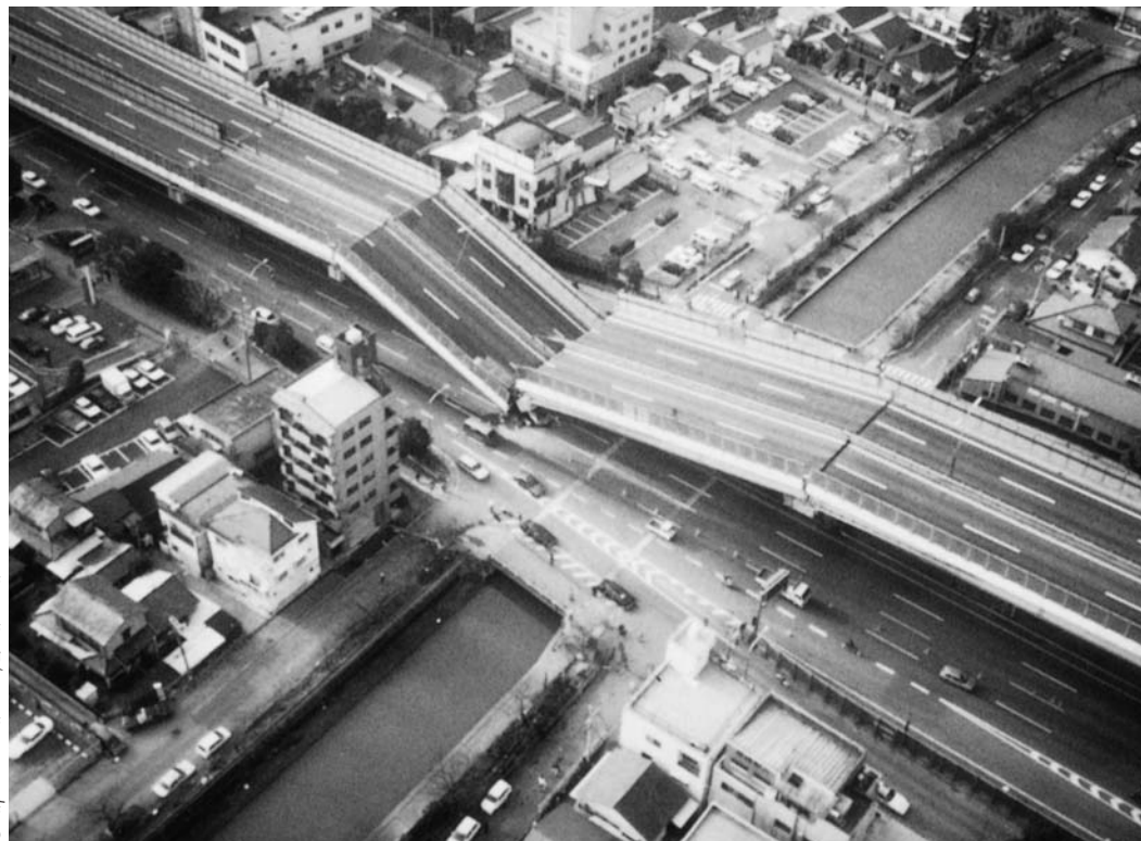
Collapsed Interstate 880, Loma Prieta, 1989
