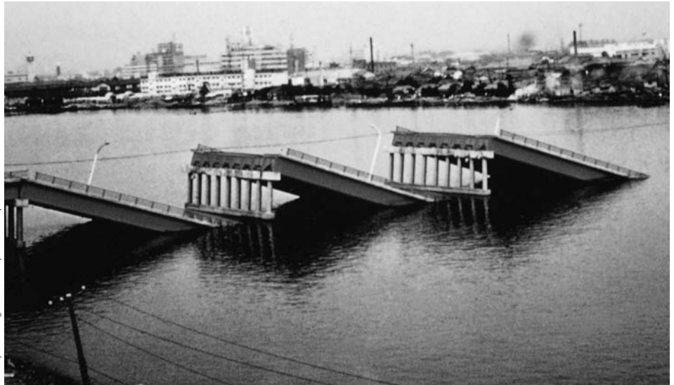
Collapsed Bridge, 1964 Japan Earthquake
