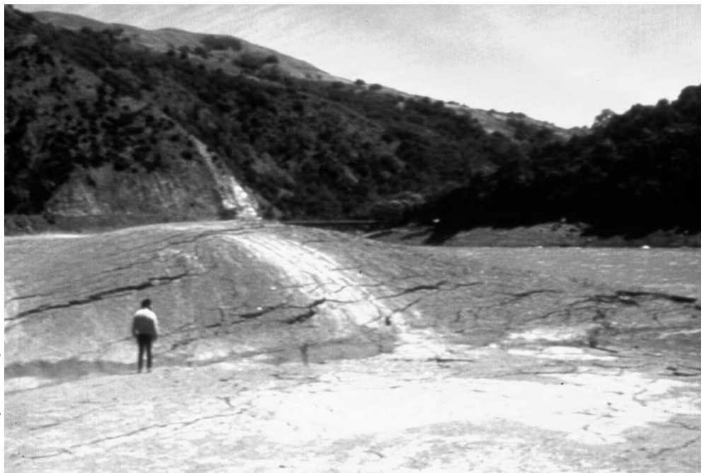
Earth dam failure, Morgan Hill, CA
